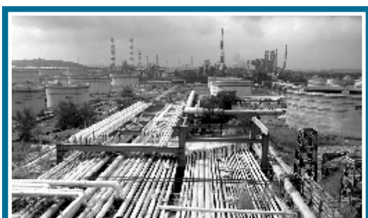
Tankage and Piping Work at MRPL Mangalore'
