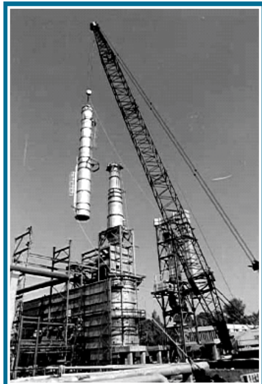
Erection of Stack in AU-IV Heater at IOCL Gujarat Refinery in the process of revamp during shutdown period
