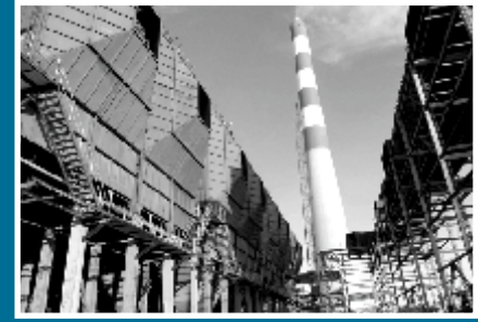
ESP at 2 X 500 MW Sagardighi STPP of West Bengal Power Development Corpn. Ltd.
