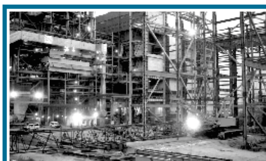
Structural works at Power House Building for Bakreswar Thermal Power Project
