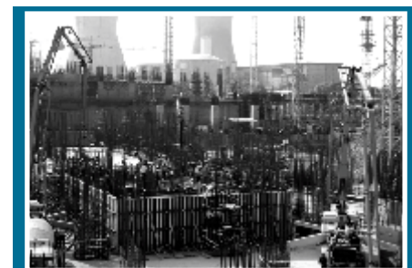
BOTI Package at Kakrapar Atomic Power Project of NPCIL
