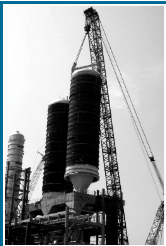
Erection of Two Coke Drums of 575 MT at DCU, CPCL, Chennai Site by Main crane 1250 MT capacity and tailing crane 550 MT
